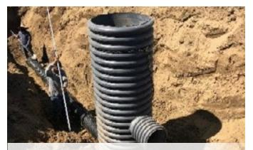
Tile drain being installed for recharge in field prior to planting. Photo provided by Glen Drown.
