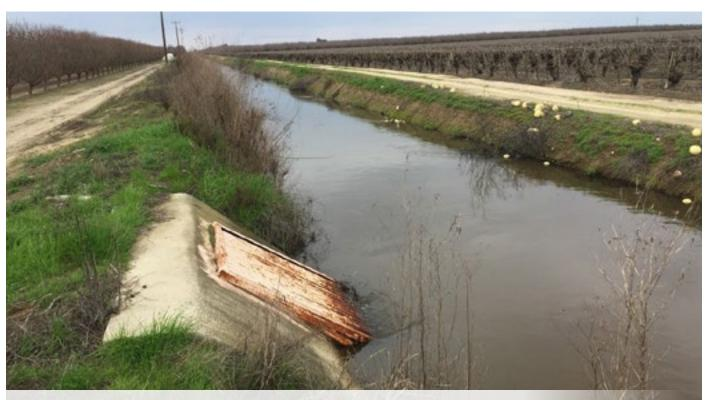
Unlined irrigation ditch in Fresno County used to convey water for recharge. Photo provided by Ladi Asgill
