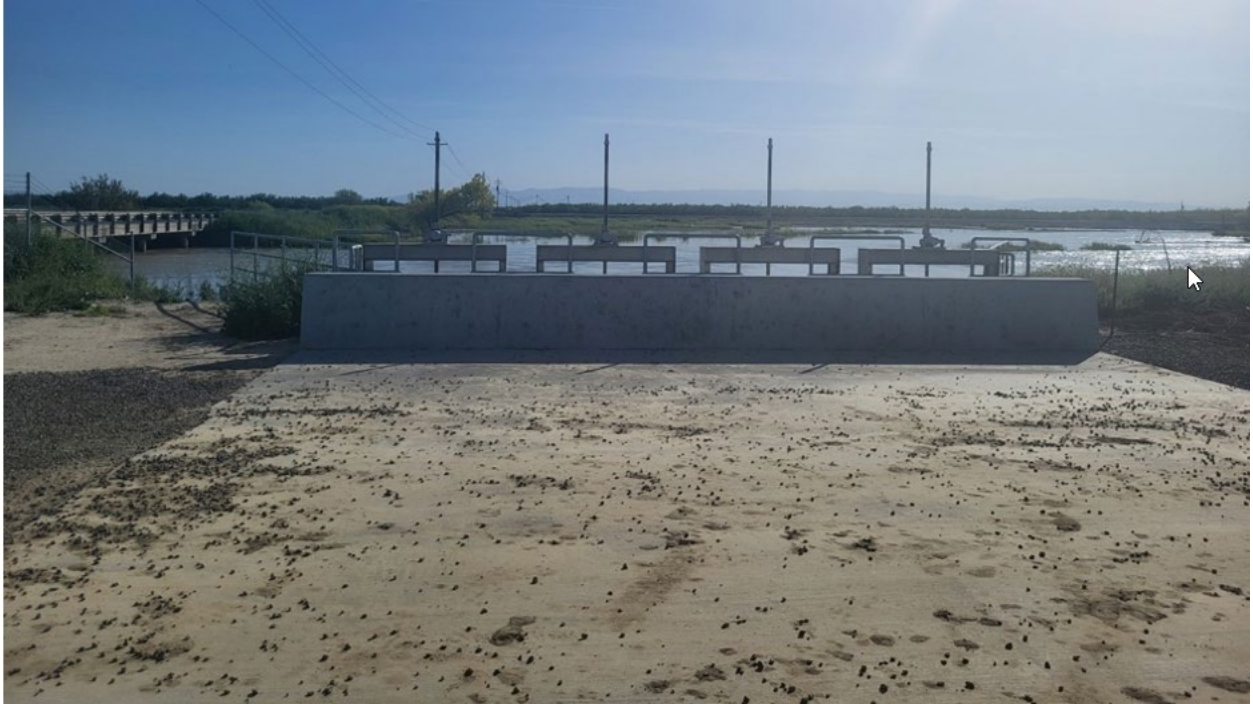
Four turnout gates on the Kings River diverting water into the Terranova Ranch canal system.
