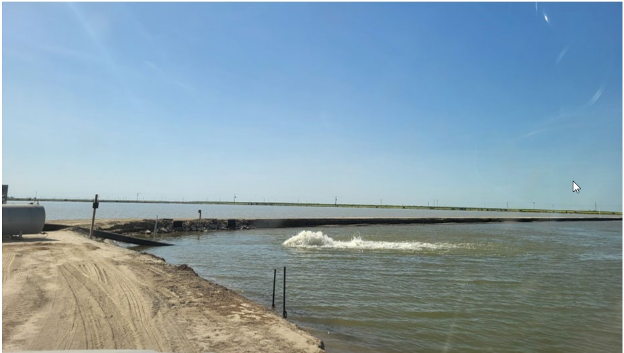
Two of three on-farm recharge unlined recharge basins, each with storage capacity of 50–60 acre-feet. Mr. Cameron has observed a significant increase in shorebird activity in and around the recharge basins.
