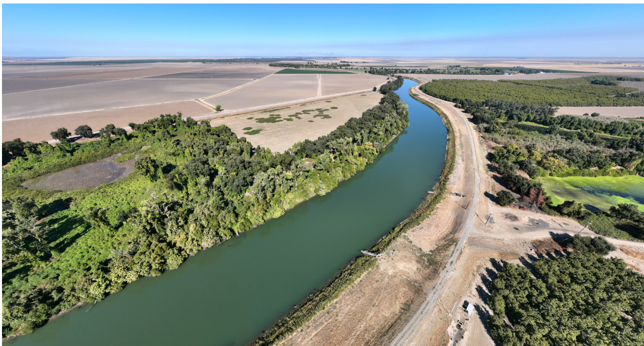
A drone view looking north over the Sacramento River in Yolo County, with the Turning Point Floodplain Restoration Project on the left side of the frame. The project is a partnership between California Department of Water Resources , River Partners , and American Rivers . The project will work on the restoration of over 1,000 acres of historical floodplain that will provide flood protection and enhance and expand critical habitat for fish and wildlife. Photo taken October 18, 2023. Fred Greaves / California Department of Water Resources.
