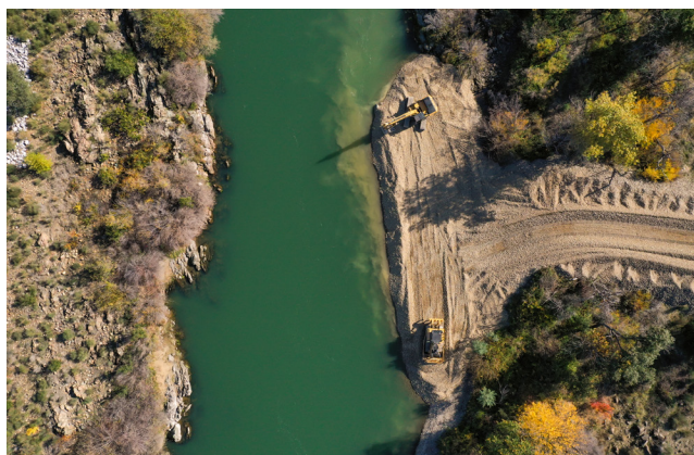
Gravel augmentation project to improve spawning conditions for Chinook salmon in the Sacramento River. Photo credit: Sacramento River Settlement Contractors.
