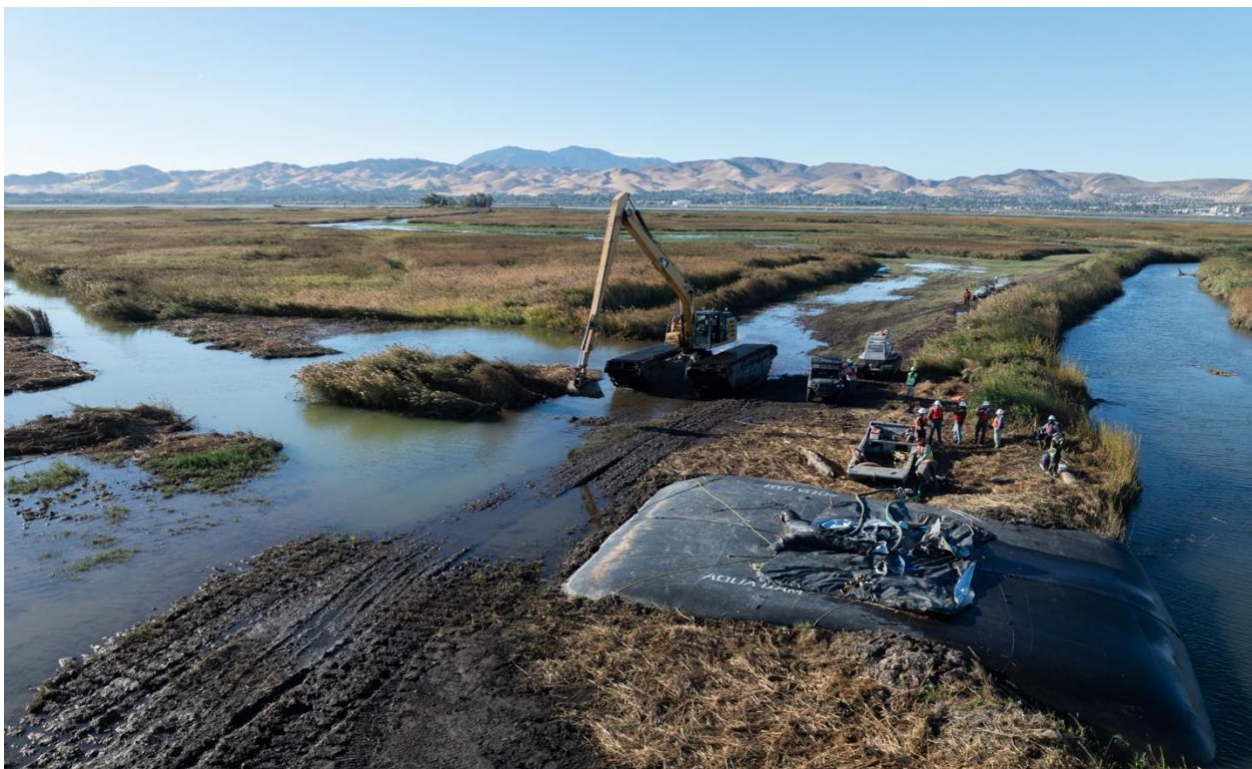
A drone view of an Aqua Dam being removed at Chipps Island Tidal Habitat Restoration Project implemented by DWR. This project will restore tidal hydrology to Chipps Island, converting previously managed wetlands to benefit native fish and wildlife species in the Sacramento-San Joaquin Delta, near Pittsburg, California. Photo taken October 2025. Credit: Andrew Nixon / DWR.
