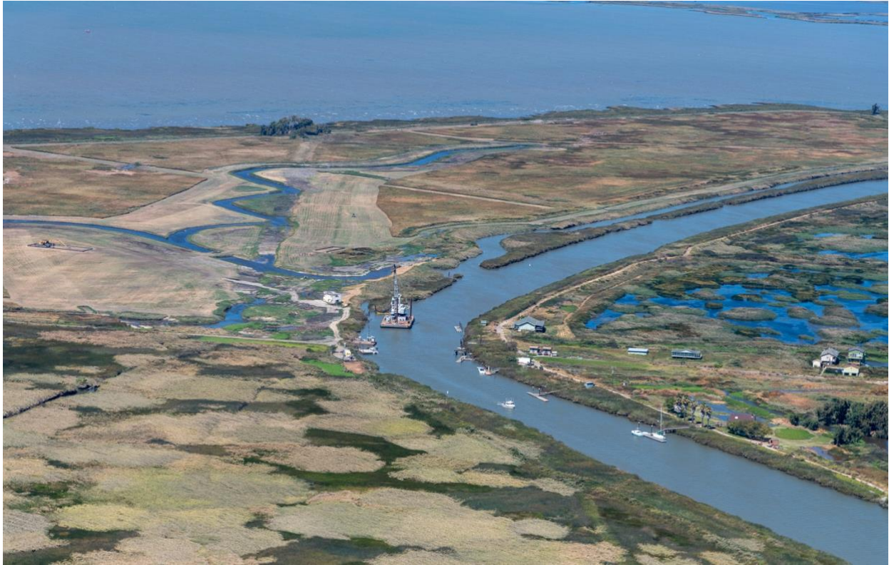
An aerial view of the Chipps Island Tidal Habitat Restoration Project, implemented by DWR. This project will restore tidal hydrology to Chipps Island, converting previously managed wetlands to benefit native fish and wildlife species in the Sacramento-San Joaquin Delta, near Pittsburg. Credit: Andrew Nixon / DWR.
