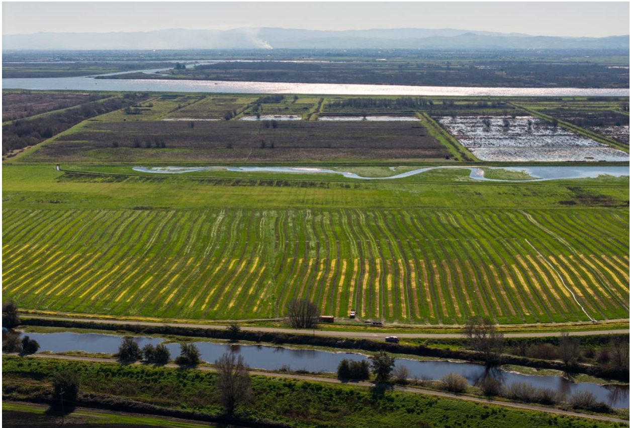
A drone image shows DWR's Twitchell Island Wetland Enhancement and Restoration Project as plant installation wraps up in February 2026. The work is creating 50+ acres of wetland habitat enhancement and about 80 acres of riparian forest and scrub-shrub habitat on one of the largest islands in the Sacramento-San Joaquin River Delta. Credit: Xavier Mascareñas / DWR
