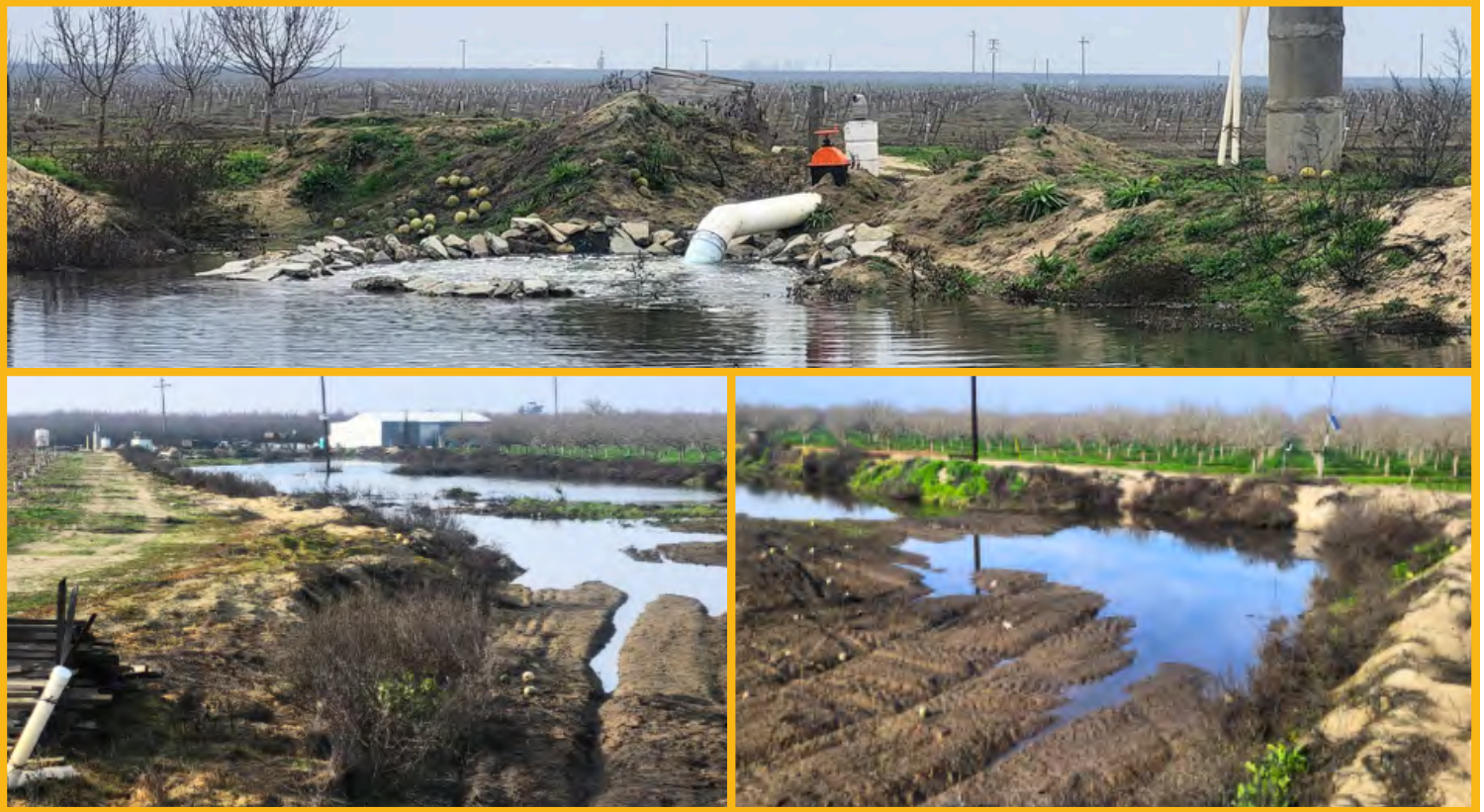
Managed aquifer recharge conducted on micro recharge basin.
