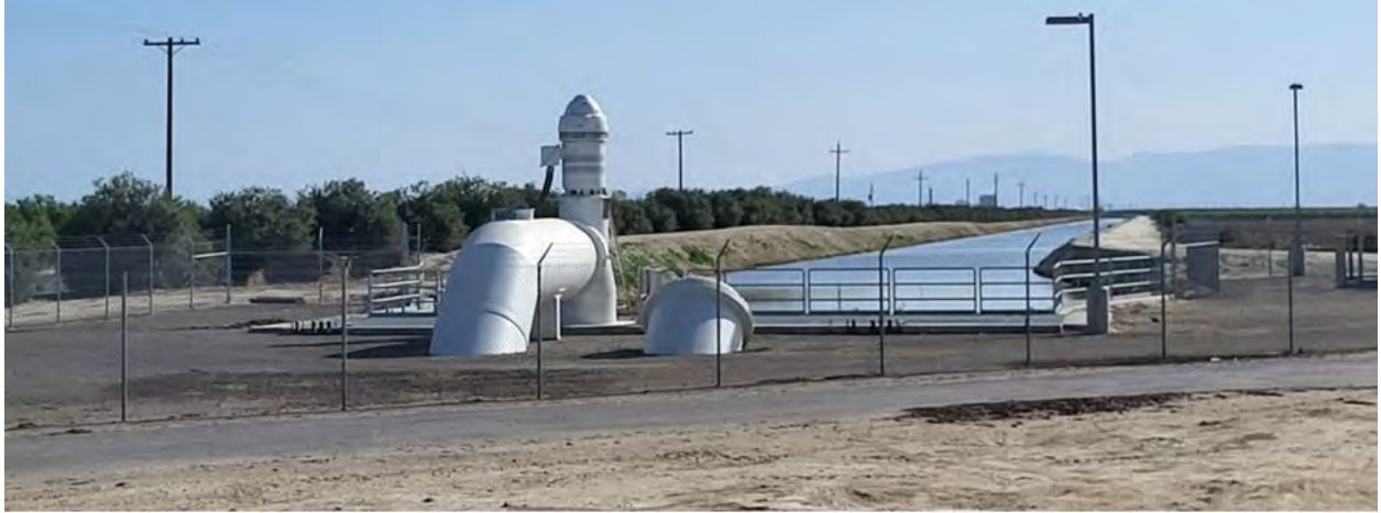
Pump used to divert water from the Kings River at peak flow levels. Maximum pump capacity of 12.5 acre-feet per hour (151 cubic feet per second).
